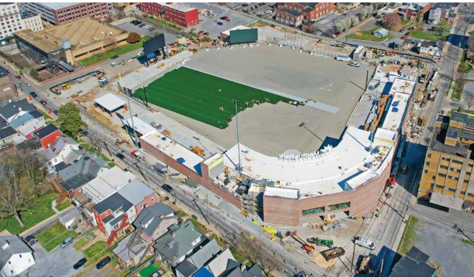
Stadium construction aerial view mid-March 2024.
